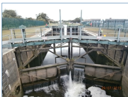
Photograph showing the upstream and middle lock gates. The paddles in the middle (ebb) gates are permanently cracked open to maintain a flow of water through the lock. This helps to disperse silt laden water drawn down from the upstream reach.
